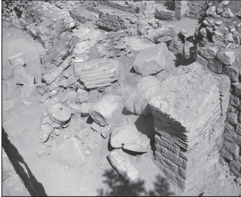
Fig. 3: Collapsed architectural elements of the wing's upper floor
